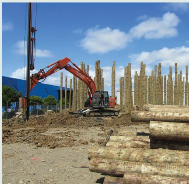
12.0m H5 TTT Uglies being pile driven as part of a foundation system for a commercial project.
