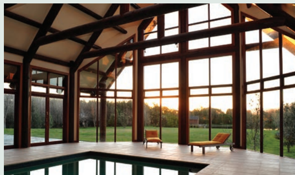
Interior view of dwelling designed by Tetrad Group Ltd architects using pre-scaled and pre-drilled UniLogs.
